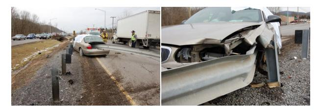
On the other hand, if the guardrail doubles over on itself after throat lock, it creates a new hazard for other approaching vehicles that may encounter the head before a maintenance crew can repair it. A doubled over guardrail after throat lock is shown below:
